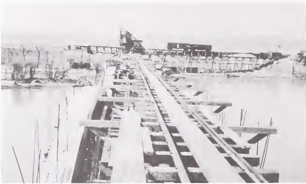
The concrete mixing plant on the north bank of the Missouri River in 1920. The ribbed arches have been completed and the deck--is about to be installed (all photographs of the construction of the Tenth Street Bridge were provided by Robert Blakeslee Photograph).
